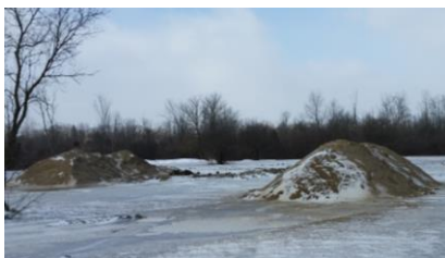
Winter installation with excavation frozen under ice/snow
